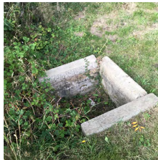
Fig. 39: Culvert invert in highways verge to south west corner of the site.
